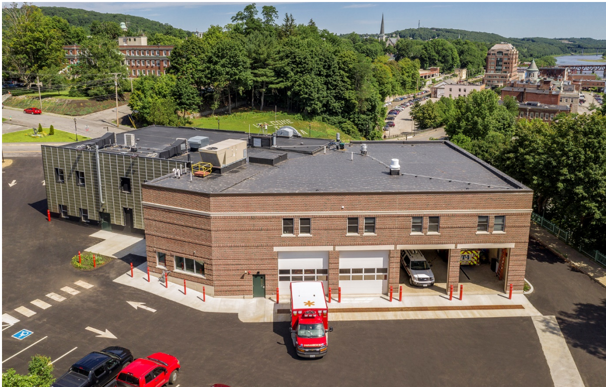
The original Classical Revival style structure underwent a major renovation, which turned its four apparatus bays into backup apparatus storage and its second floor with administrative offices, a training room, conference room, and display space for historic memorabilia.
