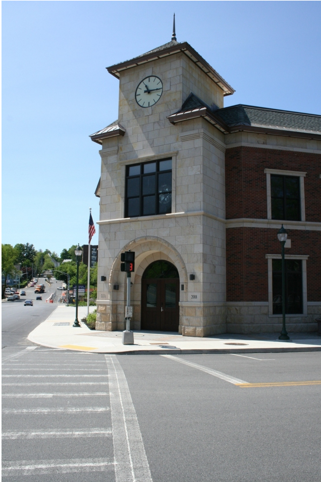
This is a state of the art fire protection facility and stands as a clear sign of the city's confidence in its future.
