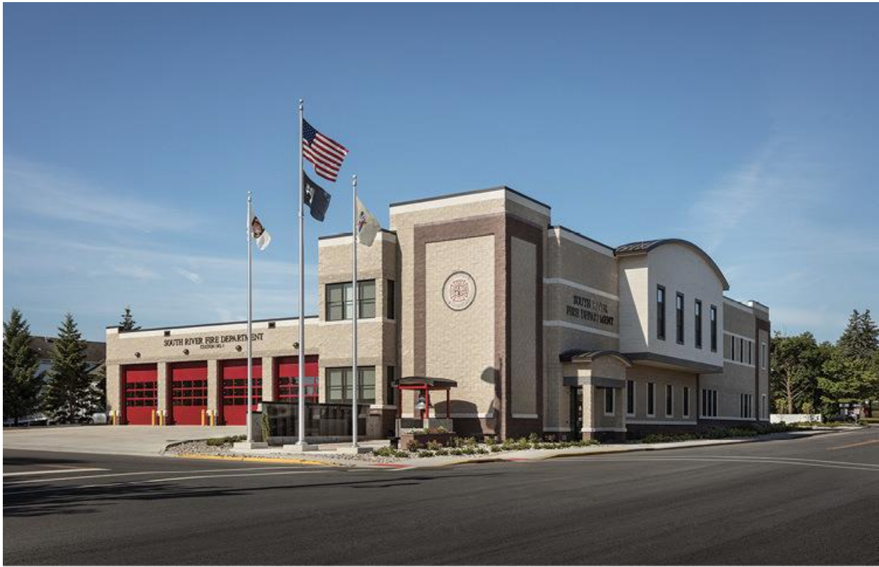
3 The Mitchell-designed station for South River is the work space for 70 volunteer firefighters.
