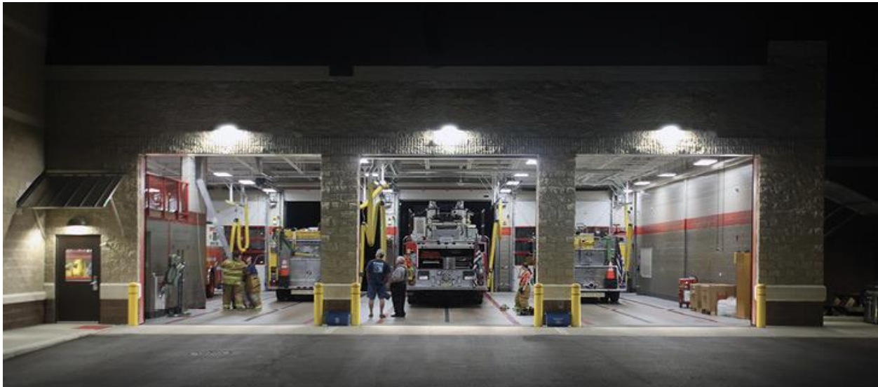
2 The rear of the South River fire station showing the back entrance to the three drive-through double-deep apparatus bays. The station also has two back-in bays.
